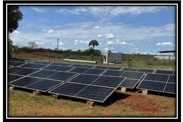
Pak Inf Batt in MINUSCA - Solar photovoltaic system low penetration system of 24 kWp deployed in 2023.
